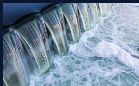
Water and Wastewater Technique
